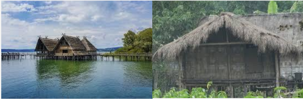
Figure 22 Mishing Tribal Houses, Assam raised on stilts and constructed using bamboo, thatch, and palm leaves.
