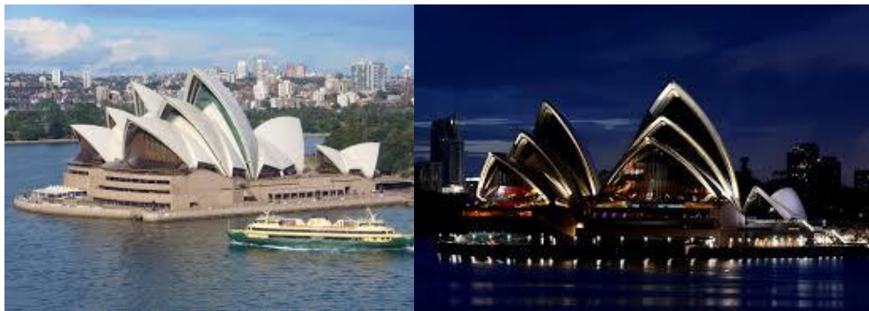
Fig 9-Sail-like roof structures resemble the billowing sails of a ship
